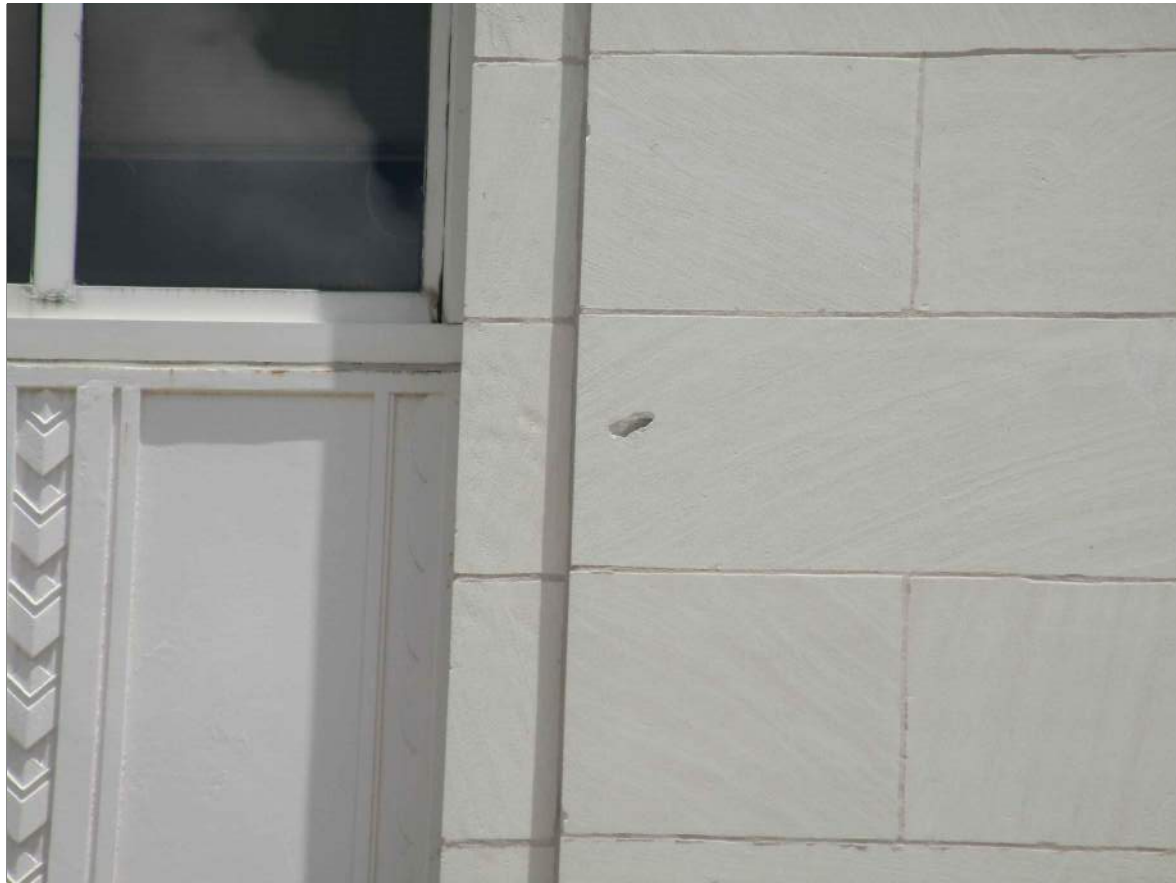
7 TYPICAL HOLE IN LIMESTONE TO BE REPAIRED
