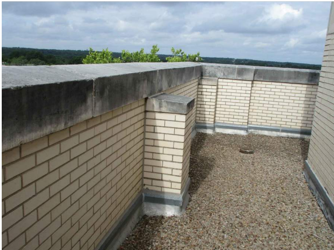
13 TYPICAL AREA OF STONE COPING TO BE CLEANED
