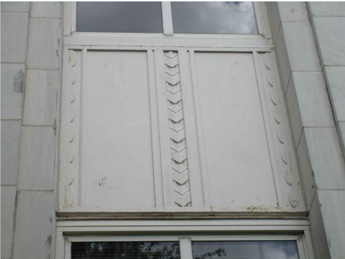
10 TYPICAL AREA OF DECORATIVE METAL PANEL TO BE REPAINTED
