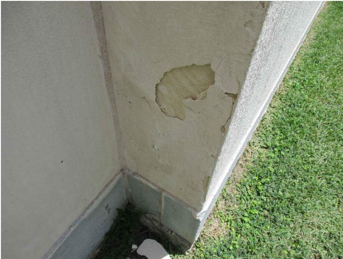
6 TYPICAL AREA OF SPALLED LIMESTONE COATING TO BE REPAIRED
