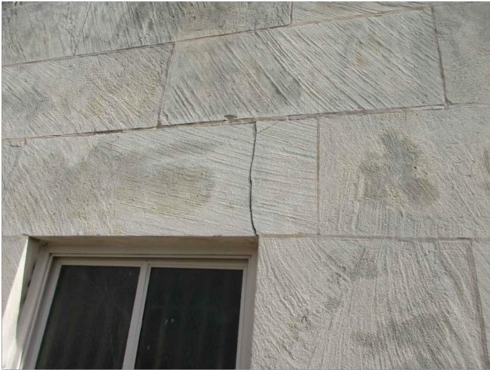
2 TYPICAL CRACK IN LIMESTONE TO BE REPAIRED
