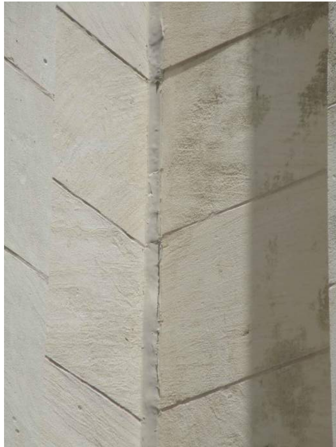
8 TYPICAL SEGMENT OF MORTAR JOINT TO BE REPAIRED
