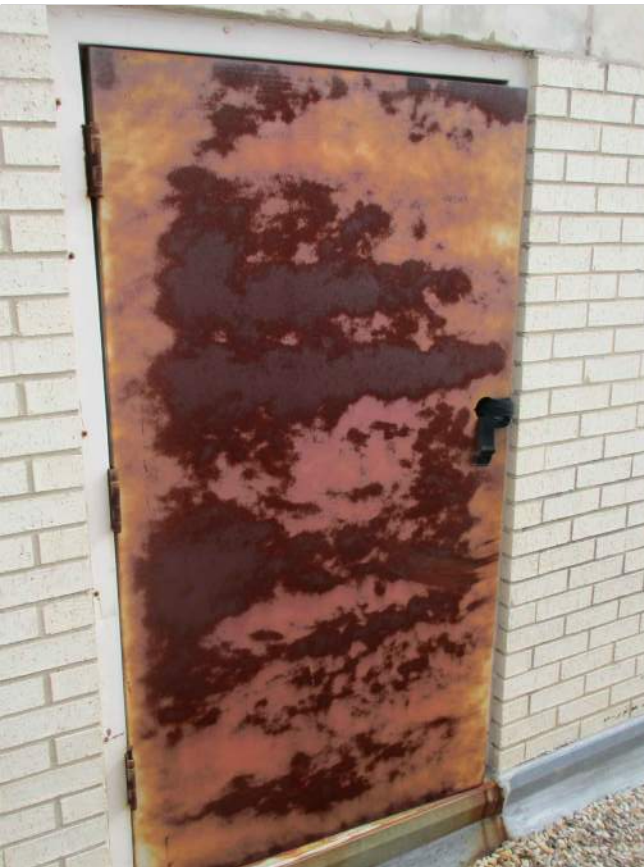
9 TYPICAL EXTERIOR DOOR TO BE REPLACED
