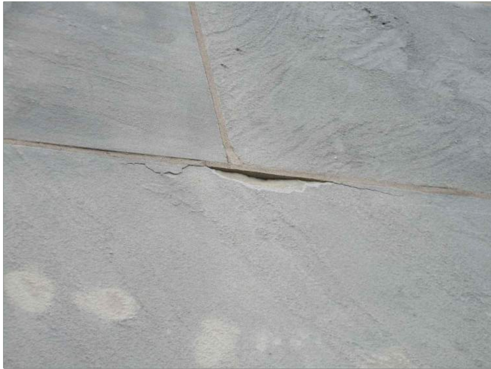
3 TYPICAL AREA OF SPALLED LIMESTONE TO BE REPAIRED
