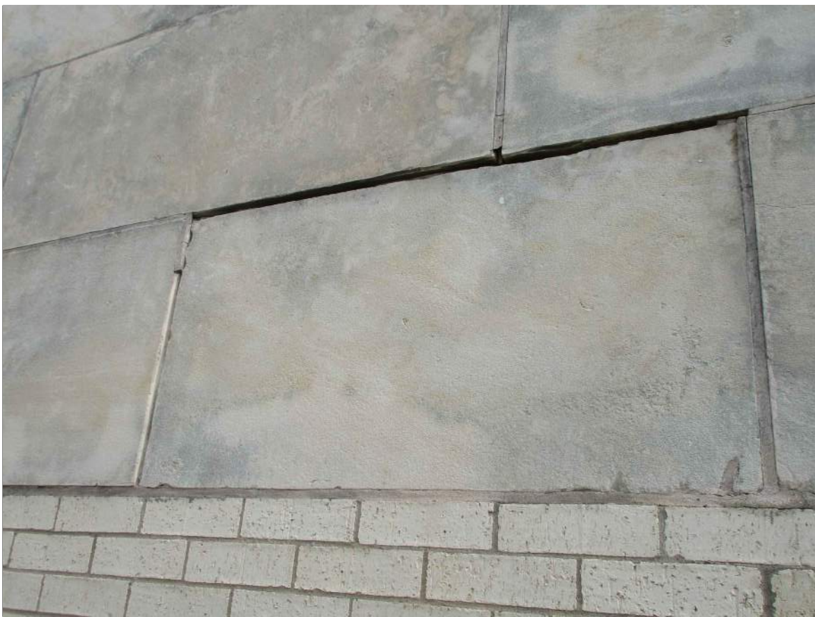
5 TYPICAL SEGMENT OF SHIFTED LIMESTONE BLOCK TO BE REPAIRED
