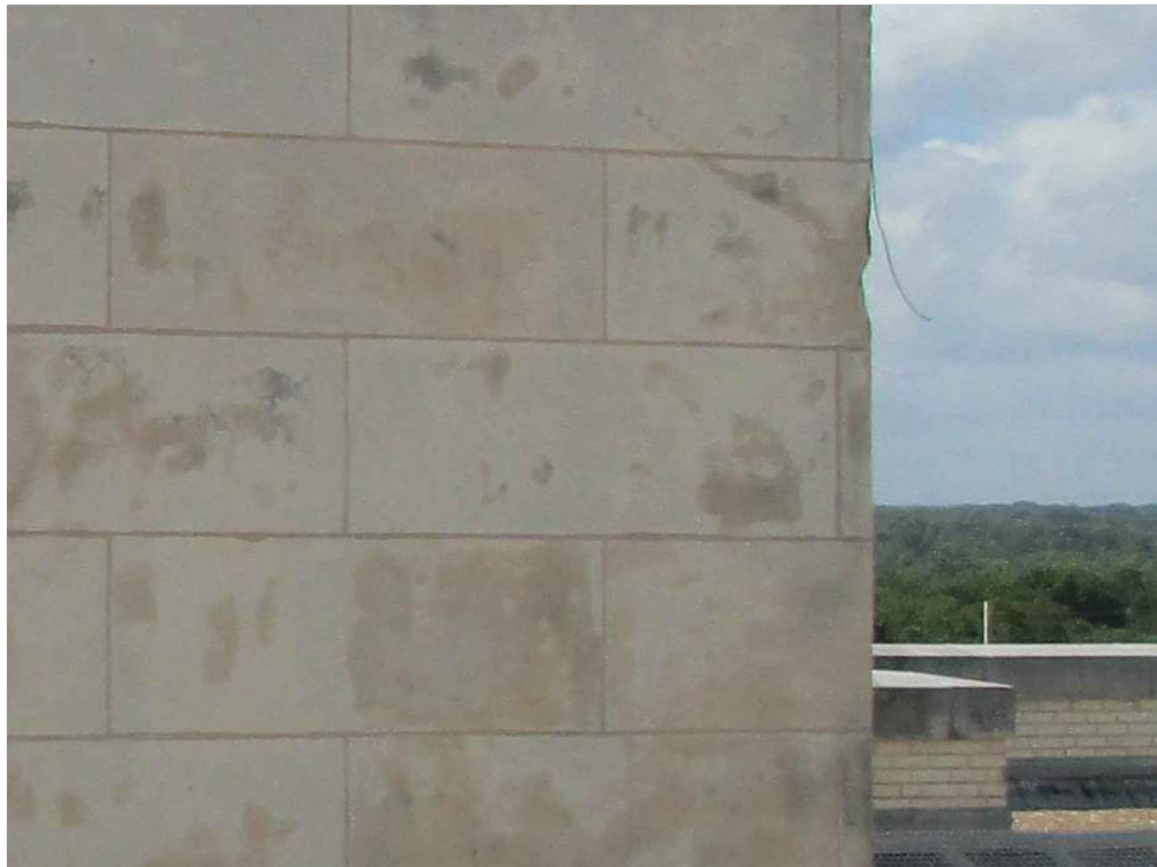
11 TYPICAL SEGMENT OF BROKEN LIMESTONE BLOCK TO BE REPAIRED
