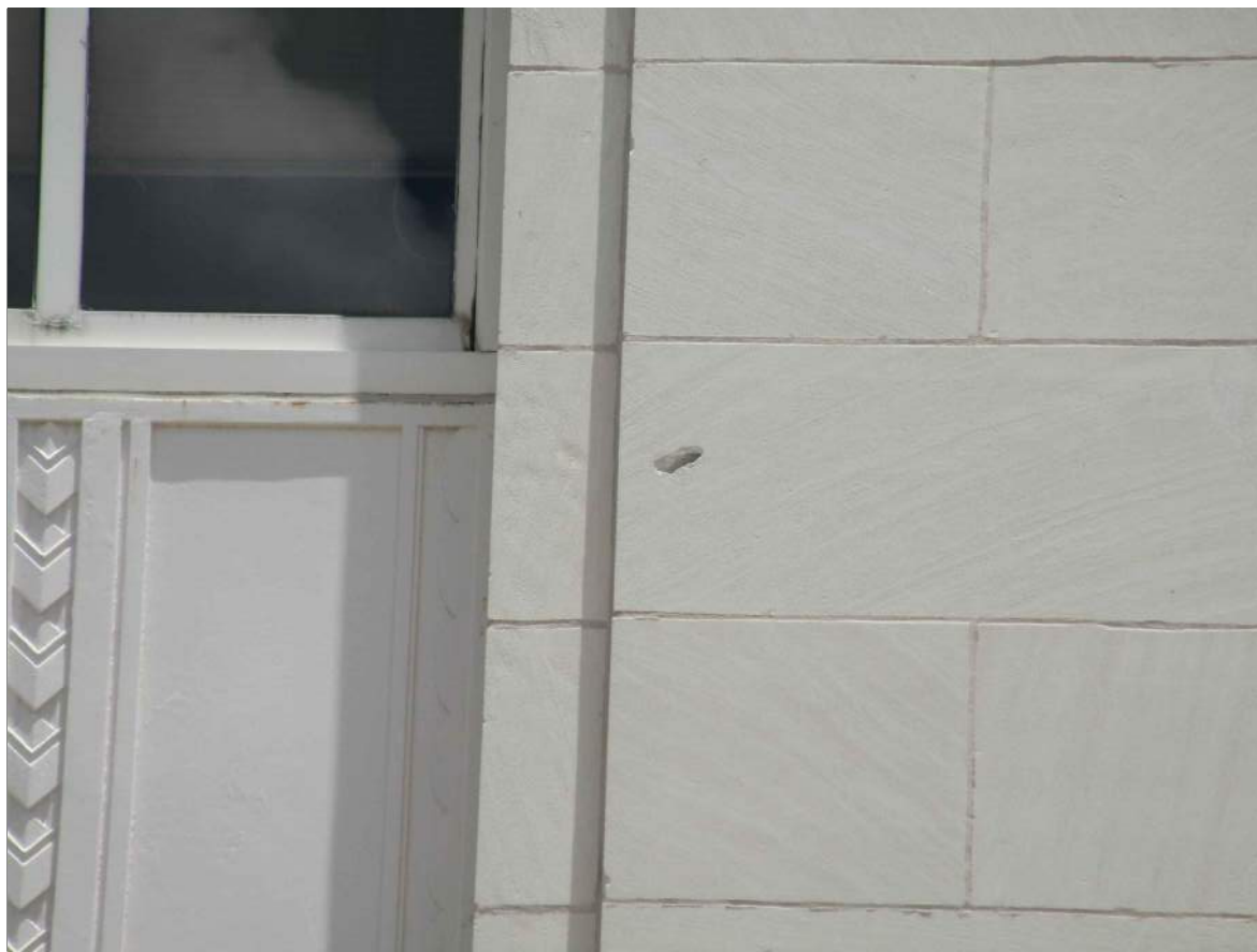
7 TYPICAL HOLE IN LIMESTONE TO BE REPAIRED
