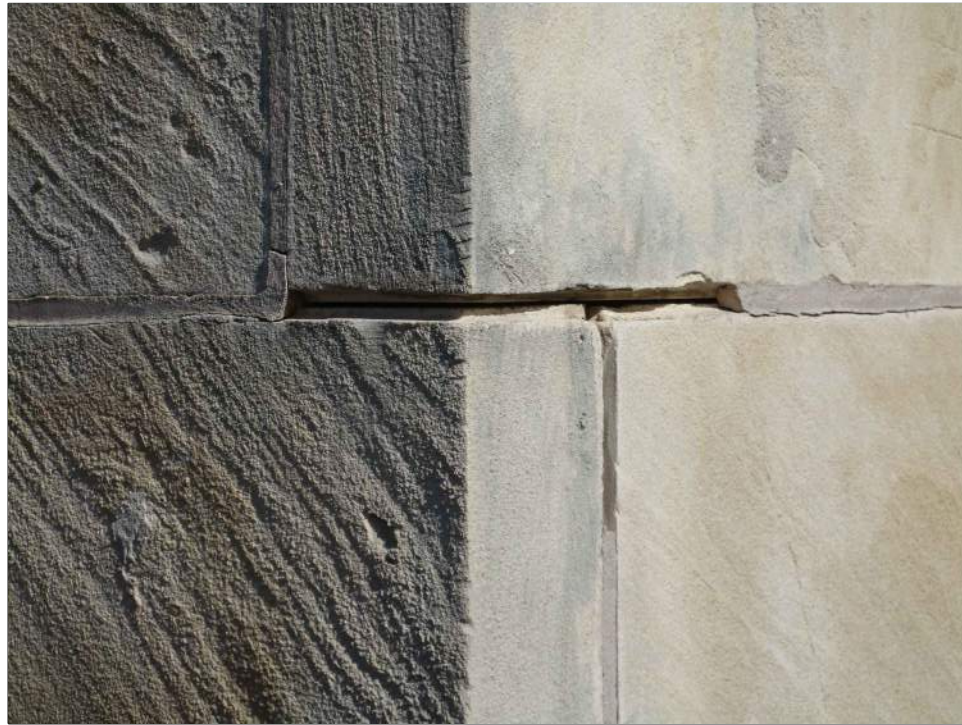
4 TYPICAL SEGMENT OF MORTAR JOINT TO BE REPAIRED
