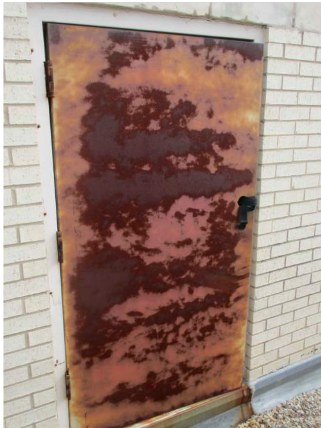
9 TYPICAL EXTERIOR DOOR TO BE REPLACED
